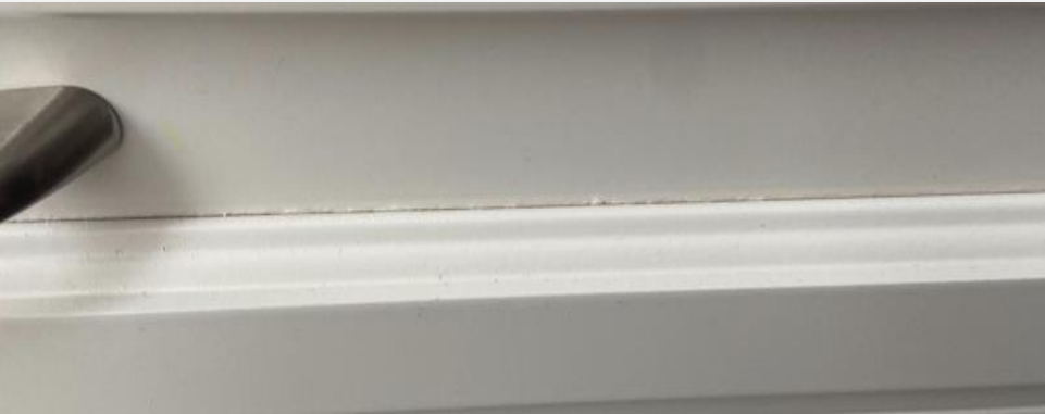
PHOTO A: Drawer front saturated by water
